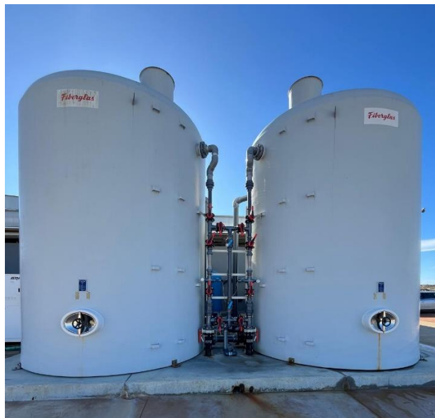
Figure 6- Exterior reservoirs (30 m 3 each) that supply the hatchery with saltwater
