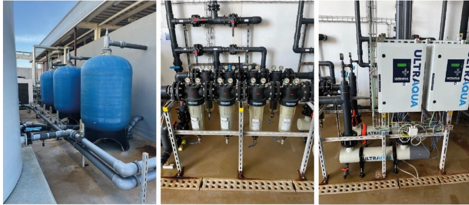
Figure 7- Exterior filtration system for the hatchery's seawater supply composed of sand filters, cartridge filters and UV lights
