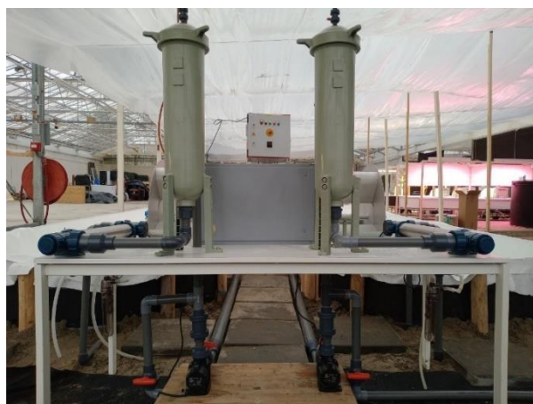
Figure 38 – Mechanical filtration system in 10,000 L raceways, showing the housing unit and filter socks ranging from 10 to 100 microns. Photo: Paulo Pereira
