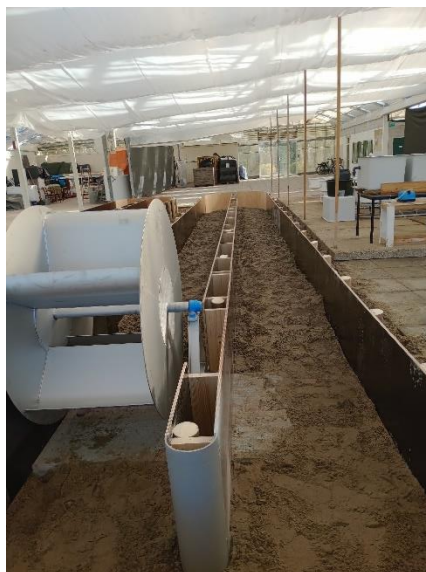
Figure 33 – Works on the ground of the raceway. Photo: Paulo Pereira
