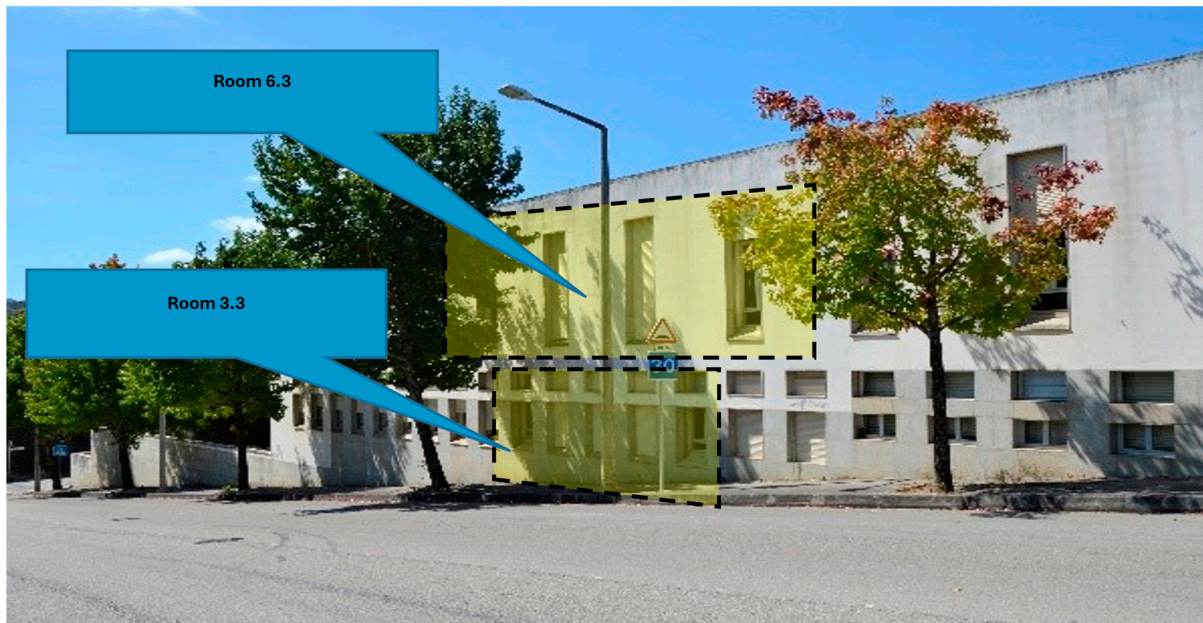
Figure 2. External façade (East oriented) of the two monitored classrooms.
