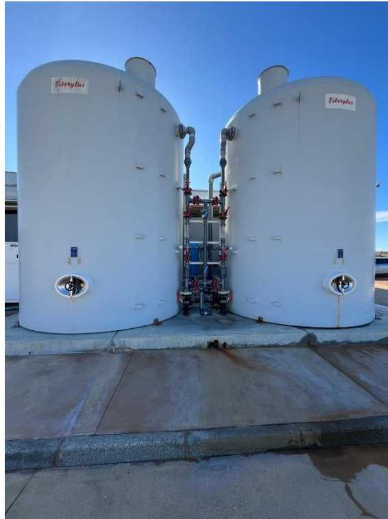
Figure 6. Hatchery reservoirs of 40,000 liters (Source: Author, 2025).
