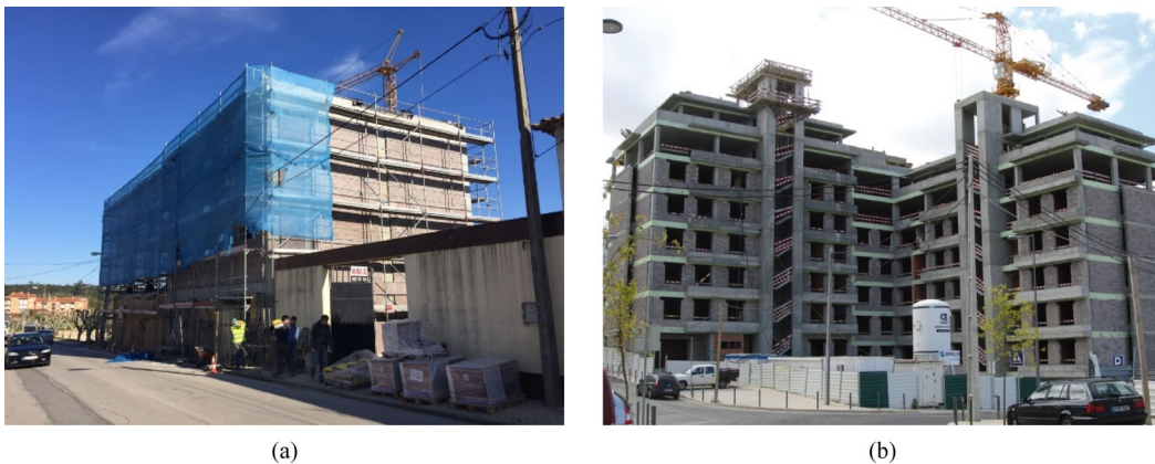
Fig. 2 Examples of buildings built with VHCB315: (a) residential and commercial 4-storey building in Soure (Portugal); (b) residential 8-storey building in Lisboa (Portugal).
