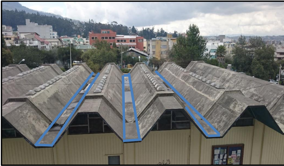
Figure 4.7 - Rainwater collection surface on the top of the Hydraulics Laboratory
