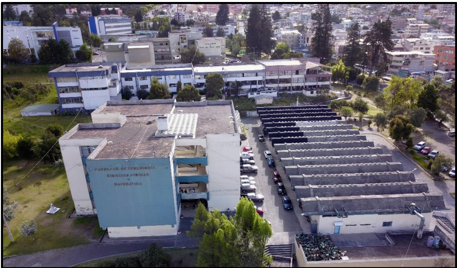
Figure 4.10 – Hydraulics Laboratory and Classroom Building Roofs Source: Author – DJI Drone
