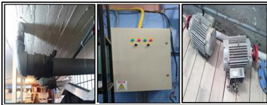
Figure 4.32 - Elevated Water Tank and Pumping System - Hydraulics Laboratory
