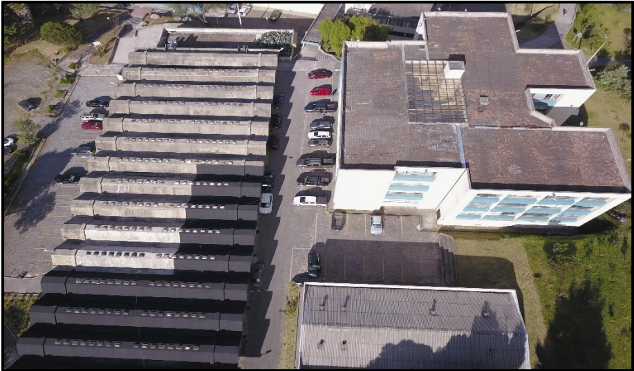
Figure 4.9 – Hydraulics Laboratory and Classroom Building Roofs Source: Author – DJI Drone
