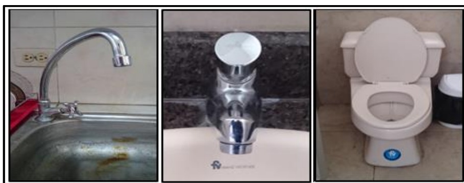
Figure 4.29 - Bathroom's devices (Women) – Third Floor
