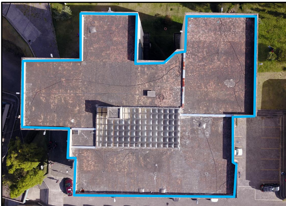
Figure 4.6 - Rainwater collection surface on the top of the Classroom Building
