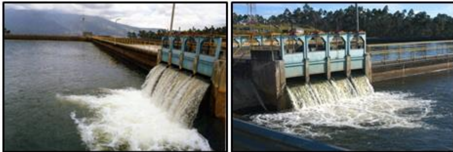
Figure 2.8 - Treatment Plants for Water in Quito
