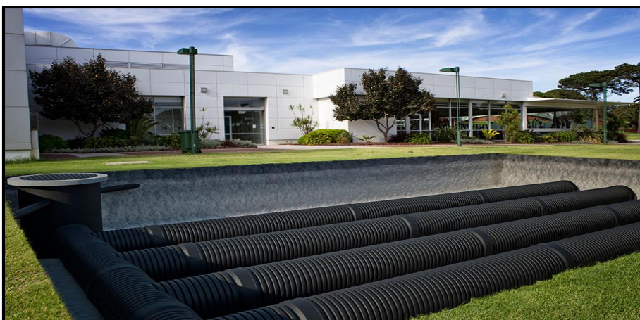
Figure 2.19 - Artificial Retention Basin
