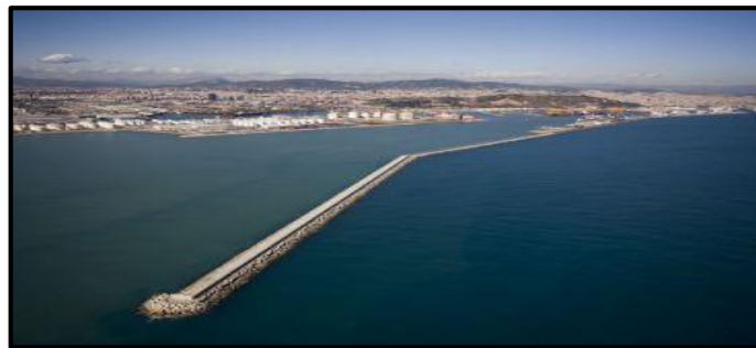
Figure 2.17 - Dyke of Barcelona's Port
