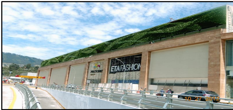
Figure 2.28 - Living wall in the Mall of Quito
