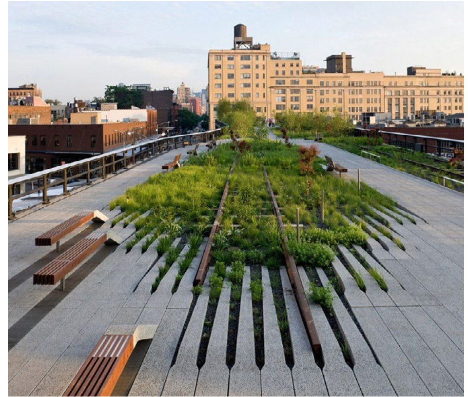
fig. 15 High Line, James Corner Field Operations, Diller Scofidio + Renfro, e Piet Oudolf.
