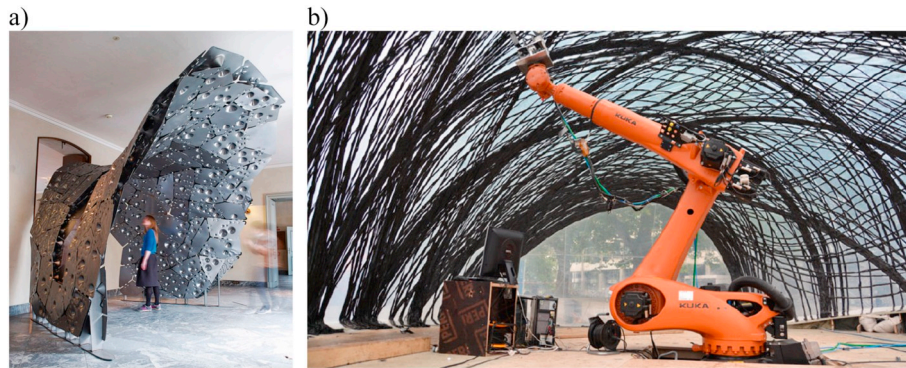
Fig. 1. a) The StressedSkins installation in exhibition at the Danish Design Museum. This is a single metallic organic structure produced by incremental sheet forming [12], b) Experimental fabrication set up of primary and secondary fiber bundles on pneumatic formwork [13].
