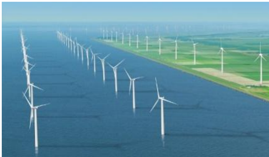
Figure 2.11 Westermeerwind wind farm, Netherlands
