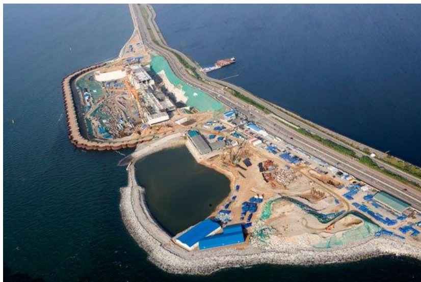
Figure 2.3 Sihwa Lake tidal power plant
