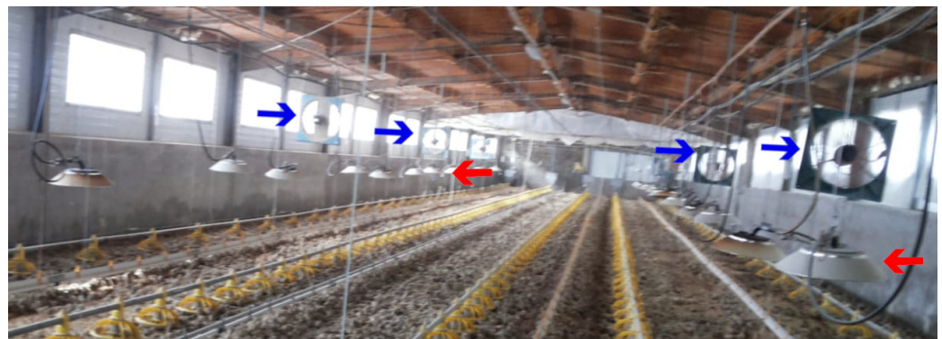
Figure 17. Poultry house with ventilation actuators (blue arrows) and heater lines (red arrows).
