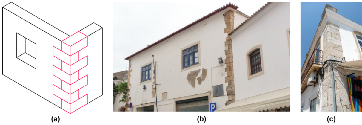
Fig. 9. (a) Traditional ashlar stone masonry quoin; (b) stone masonry quoin in Lagos, Portugal; and (c) ashlar stone masonry quoin in Vila Real de Santo António, Portugal.
