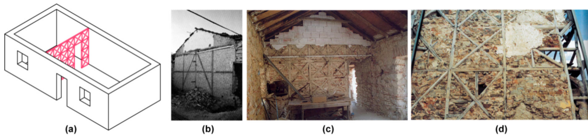
Fig. 19. (a) Traditional structural timber frame “frontal” wall; (b) “frontal” wall in Benavente, Portugal [80]; (c) “frontal” wall in Alcácer do Sal, Portugal [1]; and (d) “frontal” wall in Vila Real de Santo António, Portugal [66].
