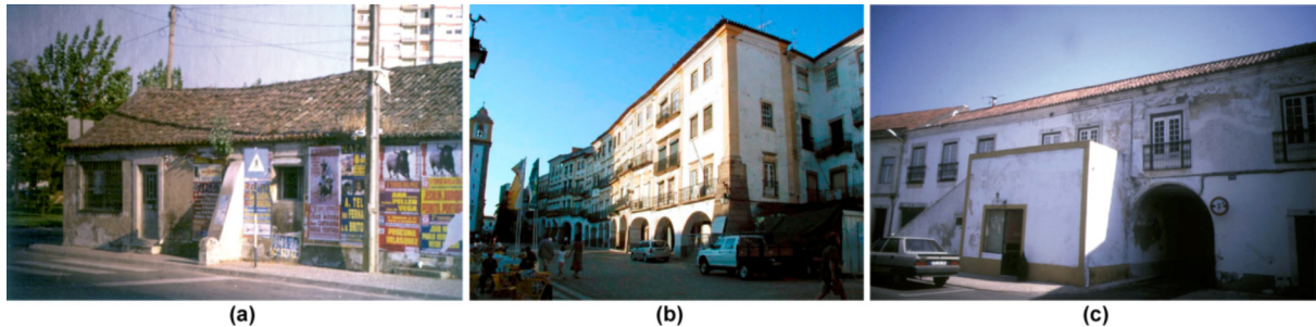
Fig. 22. (a) Butters invading the side walk in Samora Correia [1]; (b) two-floor butters in Évora [1]; and (c) external staircase in Benavente [1].
