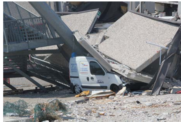
Figure 9 - Example of a collapsed cladding panel after the 2012 Emilia-Romagna Earthquake in Italy
