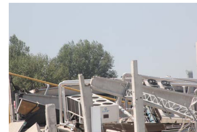
Figure 5 - Failure due to loss of support of the beam
