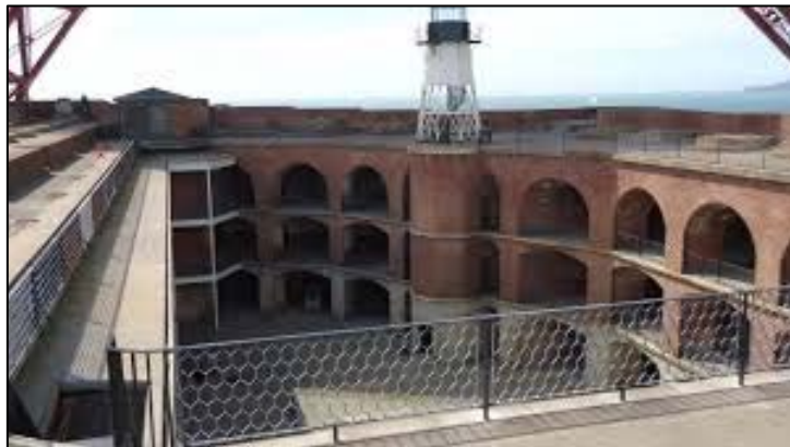
Figura 10 - Interior do Fort Point (D'Avino et al., 2012)
