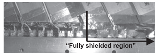
Fig. 4. Detail of the additional copper shielding placed between feedthroughs in rows above # 19. These rows will be called in the text “fully shielded region”. Note that all cells are equally shielded: the only difference is this extra copper shielding of about 2 cm length.
