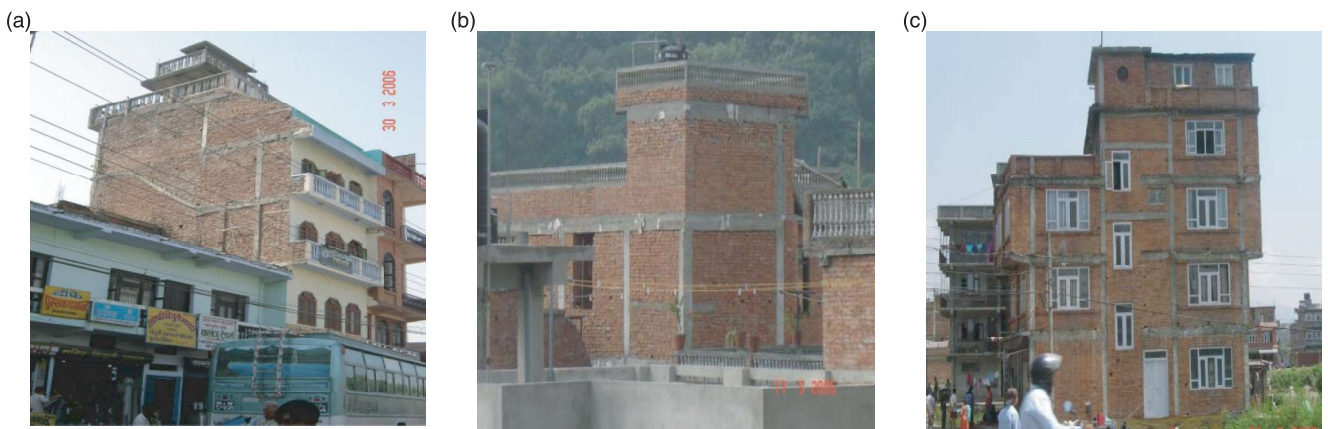
Figure 5. (a) Column starting from fifth storey; (b) Missing column in top storey; and (c) Missing beam (Marhatta et al. 2007)
