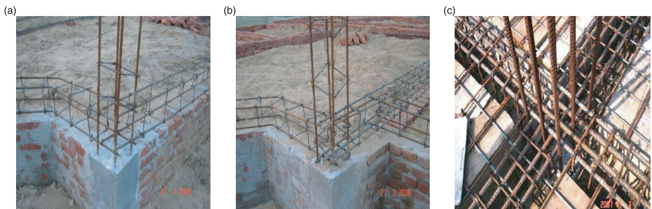
Figure 2. (a) No anchorage of beam bars in column; (b) Beam reinforcement hooking into column reinforcement; and (c) No stirrups in beam-column joint (Marhatta et al. 2007)
