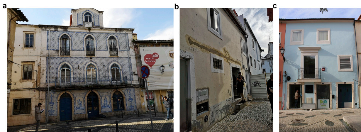
Fig. 2. Wall façades' openings: (a) Regular layout of a principal façade wall openings facing a square; (b) irregular layout of a secondary façade wall facing a minor street; and (c) latter intervention compromising the regularity of the layout of the openings.
