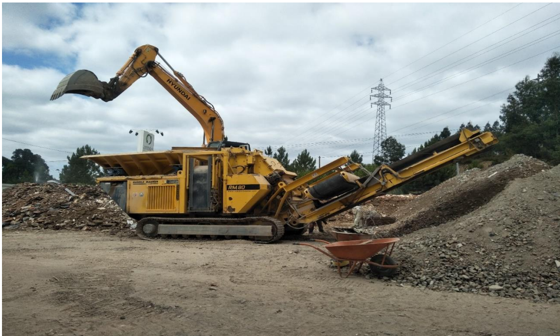
Figure 1.1 - Process of recycled aggregate
