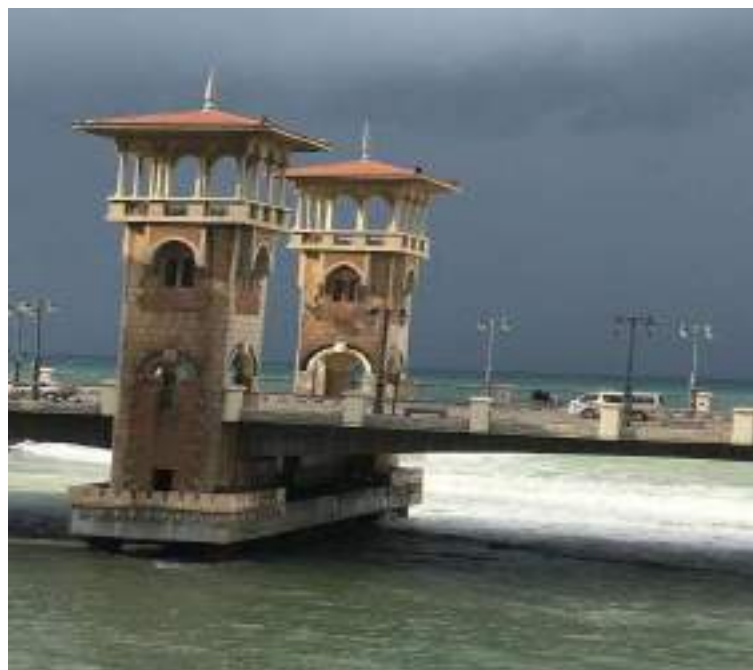
Figure 7 – Towers of Stanley Bridge
