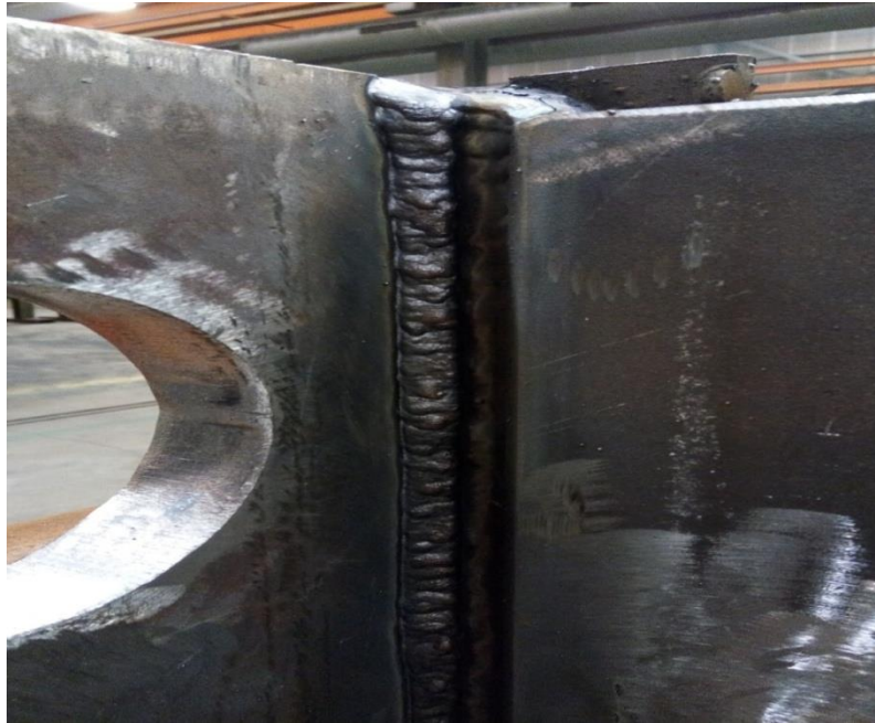
Figure 53: Flux cored arc welding (Elctrofer Group, 2017)
