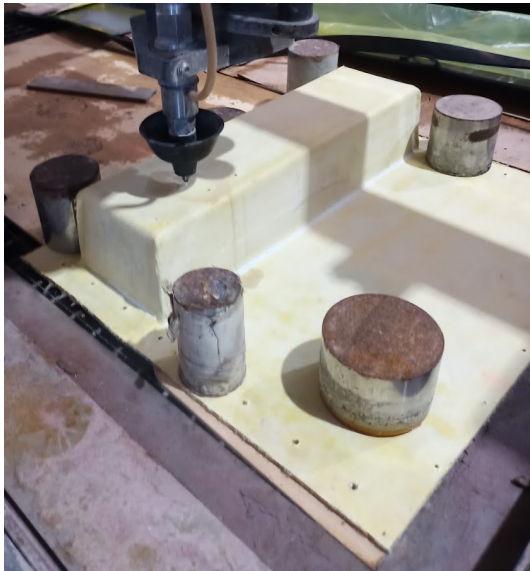
Figure 7.9: Waterjet cut HV connector openings
