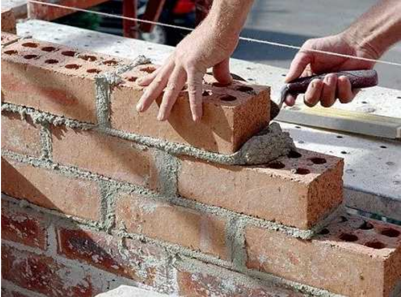
Figure 34 Locked rigging units placed on a rope for structural masonry ( http://www.arkiplus.com/mamposteria )
