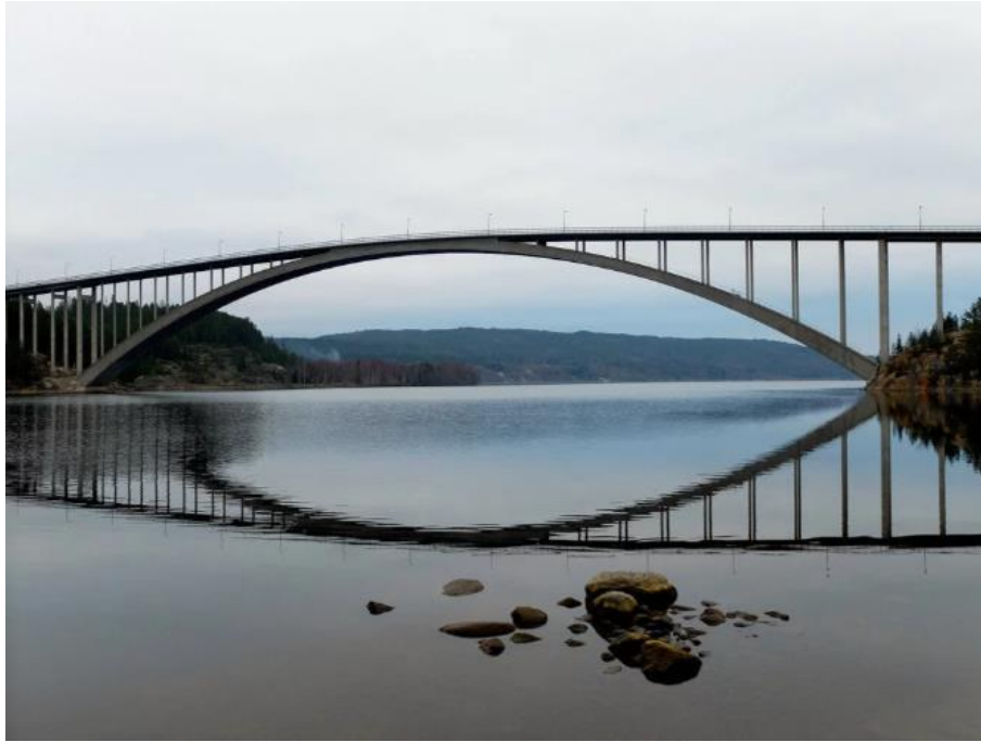
Figura 7: Ponte Sandö – Suécia ( https://en.advisor.travel/poi/Sando-Bridge-9017 )
