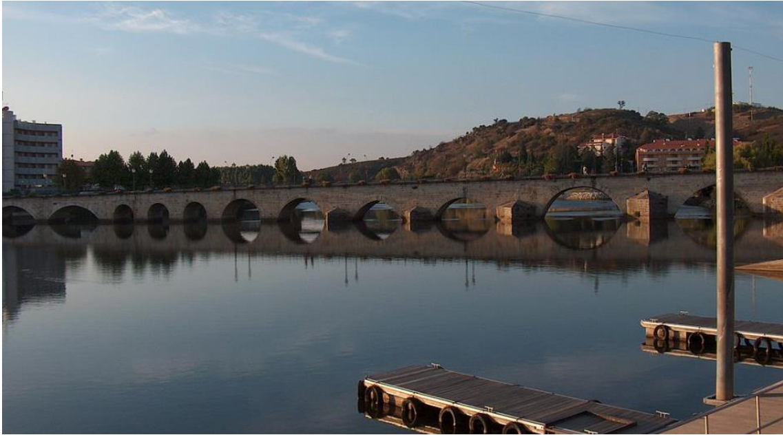
Figura 17: Ponte de Mirandela, Portugal (Wikipedia)
