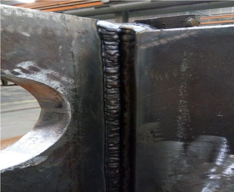
Figure 52: Flux cored arc welding (Elctrofer Group, 2017)
