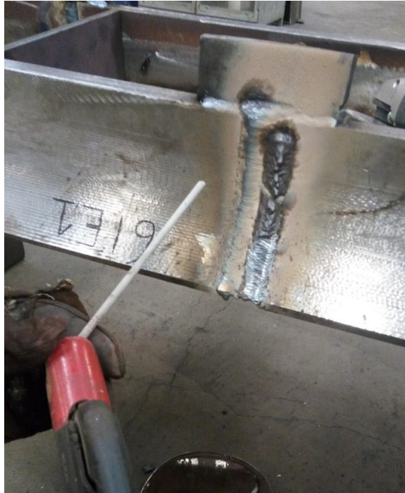
Figure 55: Shielded metal arc welding process (Electrofer Group, 2017)
