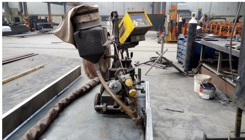
Figure 54: Submerged Arc welding process (Elctrofer Group, 2017)
