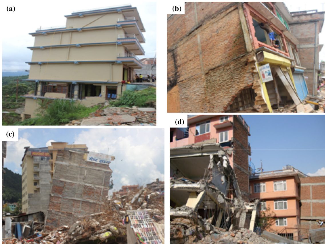
Fig. 9 a RC building in stepped foundation with partial damage. b Building tilted with column failure due to stepped foundation. c Large displacement in foundation led tilting of building constructed
