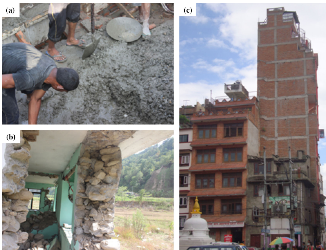
Fig. 4 a Common concrete mixing method with high water cement ratio in residential constructions. b Damaged wall due to improper binding on rounded aggregates in Melamchi (Sindhupalchowk). c An example of slender structure in Kathmandu metropolitan city
