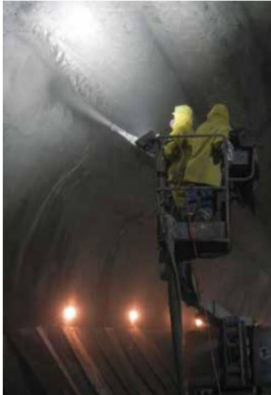
Figure 2.1: Shotcrete for rock support with manually controlled nozzle (taken from [23]).
