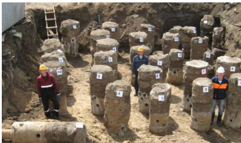
Figura 4.7 – Colunas de teste de jet grouting [45].
