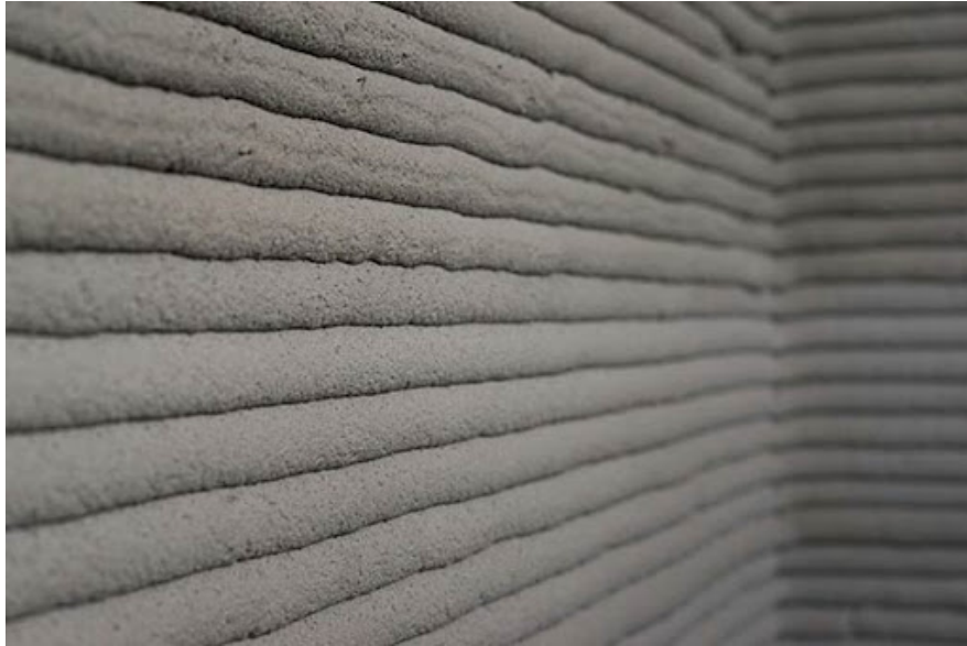
Figure 2.1: AM concrete wall [2]
