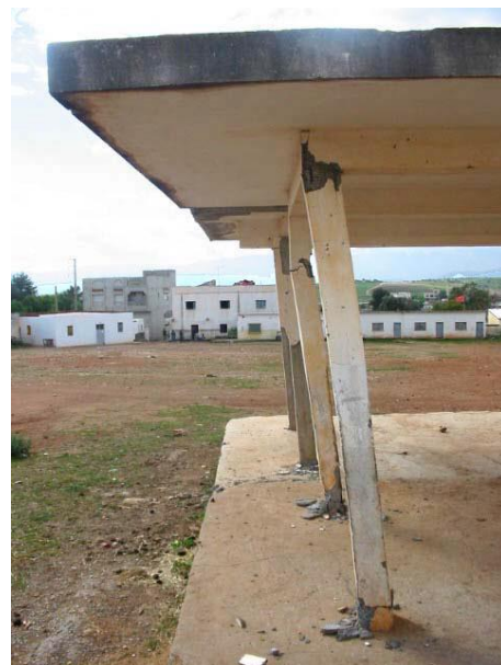
Figure 1.5: Inadequate detailing of the joints [34]
