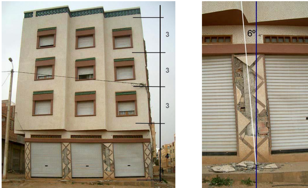
a) Behaviour of irregular structure under seismic action
