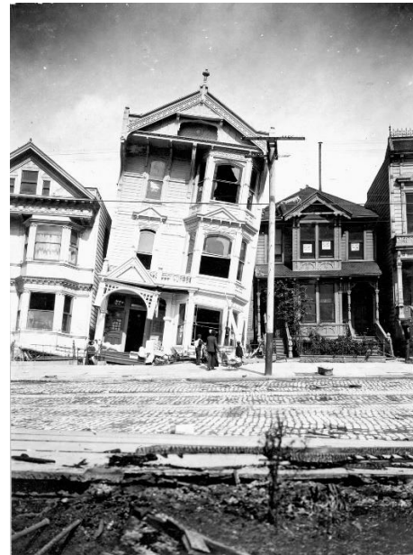
b) Soil failure
