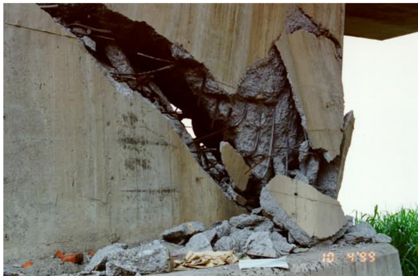
Figure 1.12: Diagonal shear crack in lightly reinforced concrete pier of the Wu Shu bridge in Taichung [39]
