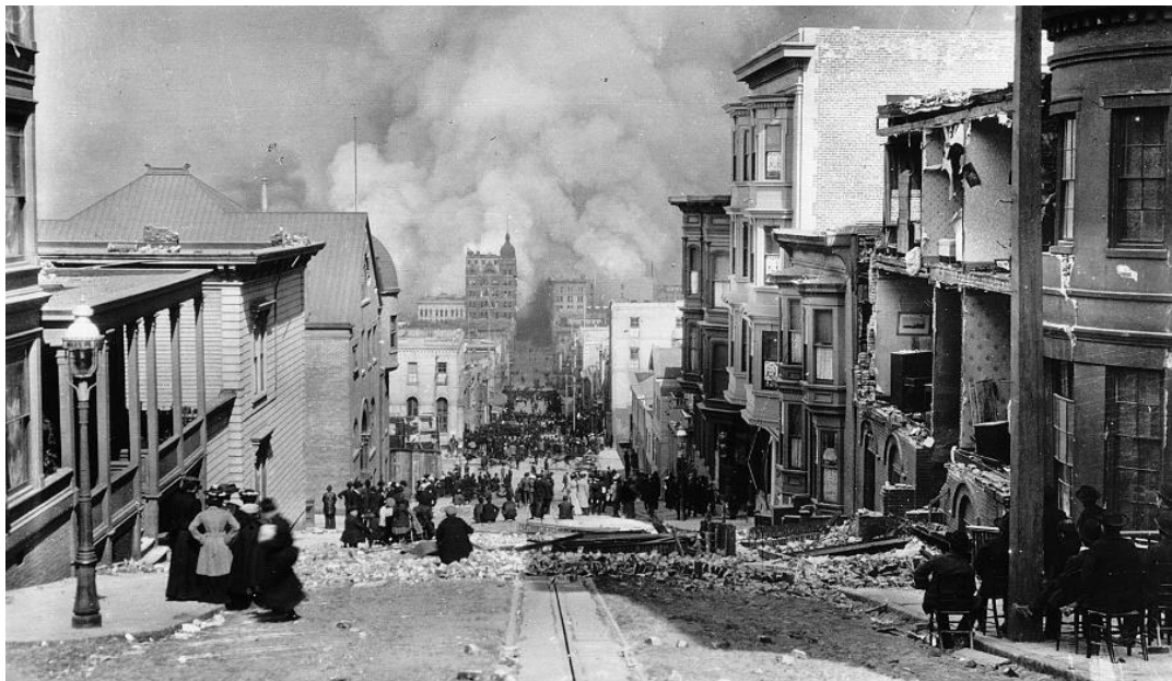
c) After Earthquake
