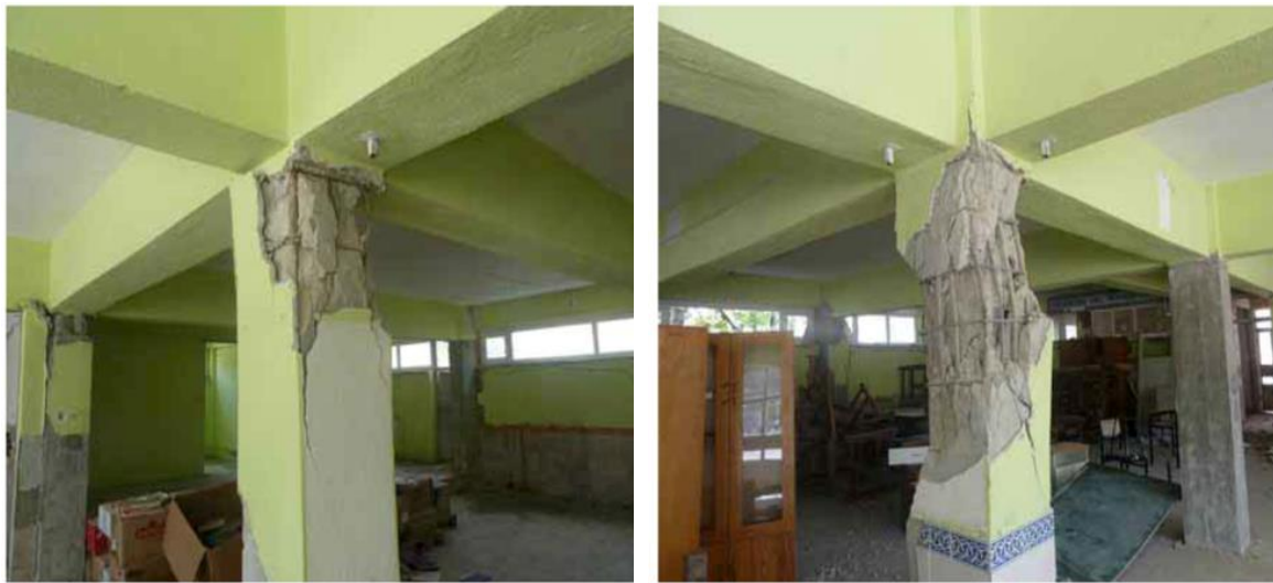
Figure 1.4: “Strong-Beam Weak-Column” failure [33]
